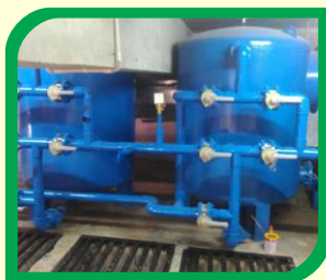
SAND & CARBON FILTER
